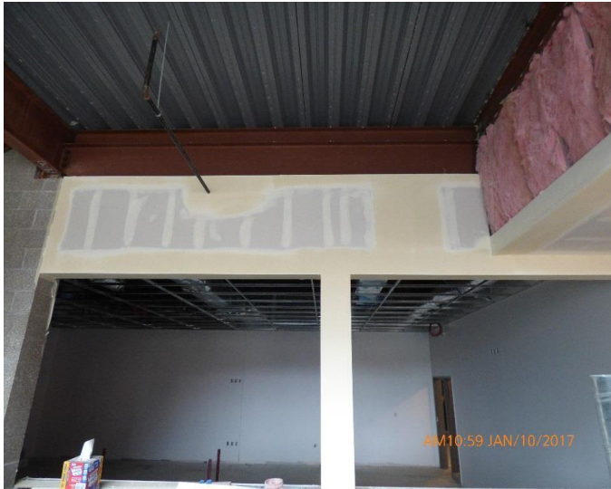
Sector 2 Drywall Soffit Prep for Paint
