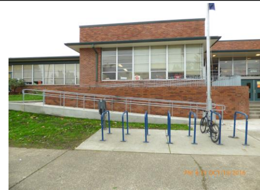
New ADA Ramp at Scott
