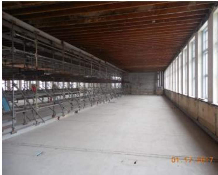
South Wing 2 nd Level – Demo Complete & Shoring Installed
