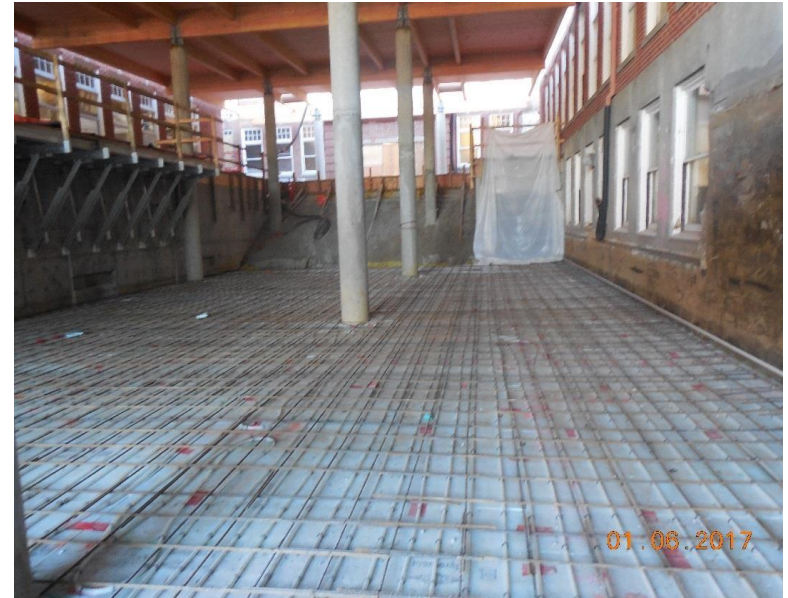
B2 Commons Ground Level - Hydronic Piping at SOG
